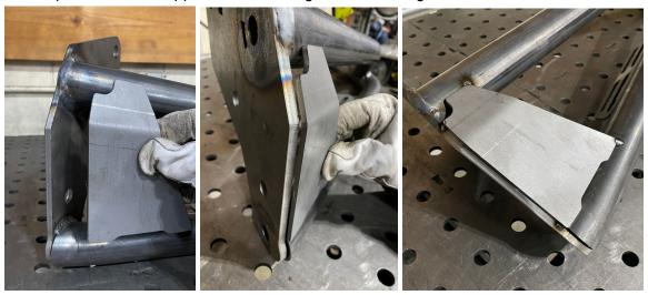
13. Fully weld the outside open corner between the formed cover and mounting bracket. Continue this weld down along the end of the upper tube and end of the top plate. (OPTIONAL: Grind welds smooth to a radius)
