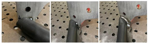
7. Take the light bracket and align the slot on it with the tab on the top of the alignment tab. The bracket should be parallel to the top surface of the wing. Put lage tacks on either end where it touches the tube. Weld over the tab/slot. Grind the weld smooth/flush with the surface.
